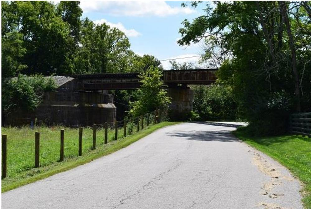
**Figure 120. The pony plate girder bridge located on Renick Street.**
