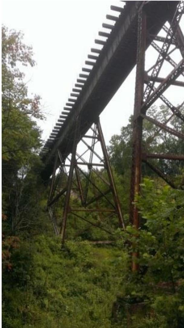
**Figure 116. Detail of the substructure and underside of the superstructure of the Howard's Creek Viaduct.**
